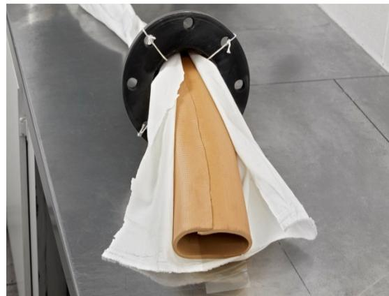
8, Pulling Tube through pipe with Cloth Liner
