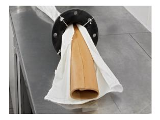
8, Pulling Tube through pipe with Cloth Liner
