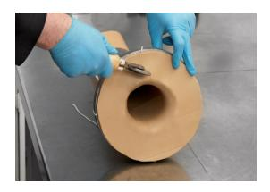
14, Placing Flange cover to Flange face
